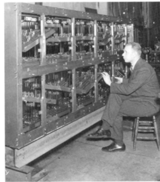
Figure 22.1 Professor John Wilbur and his mechanical computer
